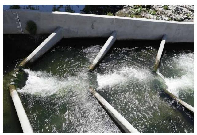
Water flows through a cement fish ladder maintained by Alameda County Water District that's along Alameda Creek in the Fremont area, as seen in 2024. The fish ladders help salmon and trout surmount man-made obstacles such as dams as the swim upstream.
